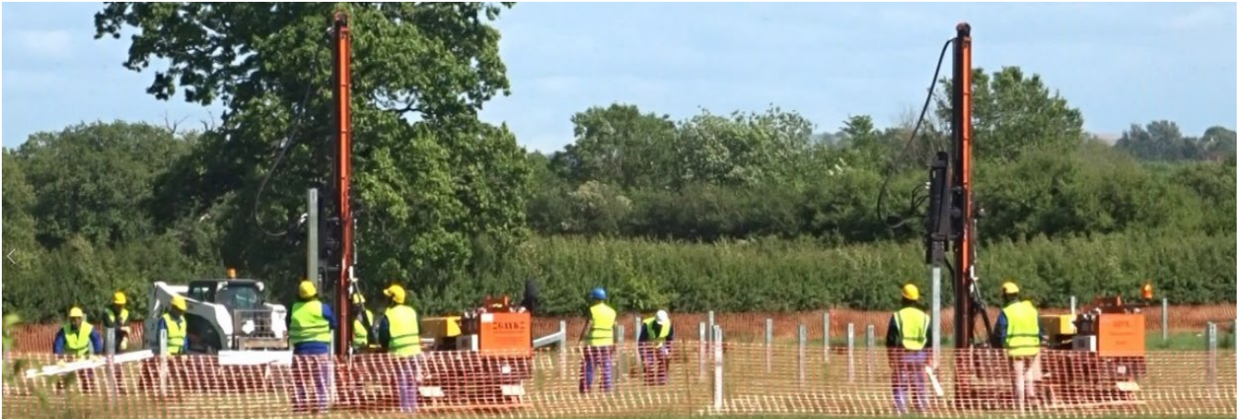
Plate 15.11: Legs being Installed
