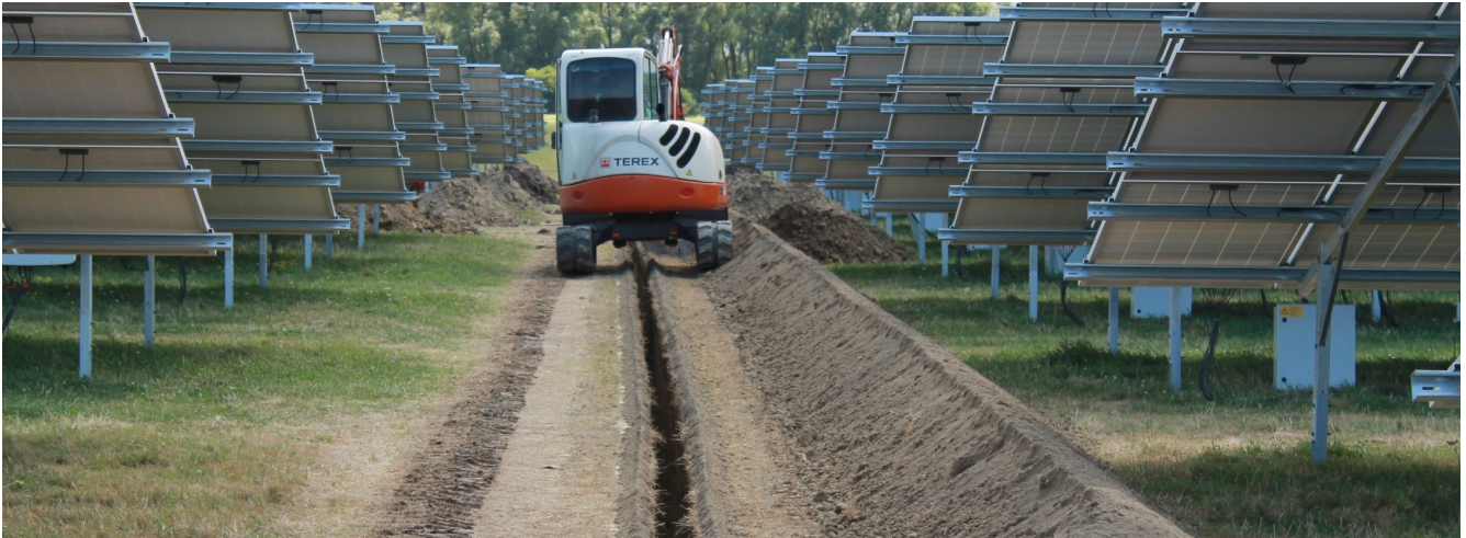
Plate 15.17: Cabling Channels during Cable Installation
